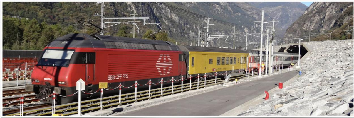
Figure 3: SBB MeWa12 Telecom Measurement Train leaving the Gotthard Tunnel at the south portal
